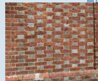
Brickwork in Flemish Bond
